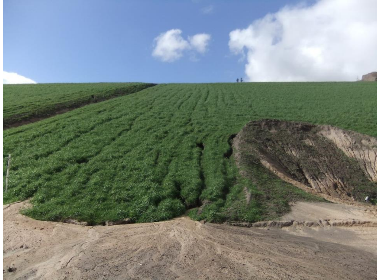
Yallourn Interim Rehab Eastern Batters
