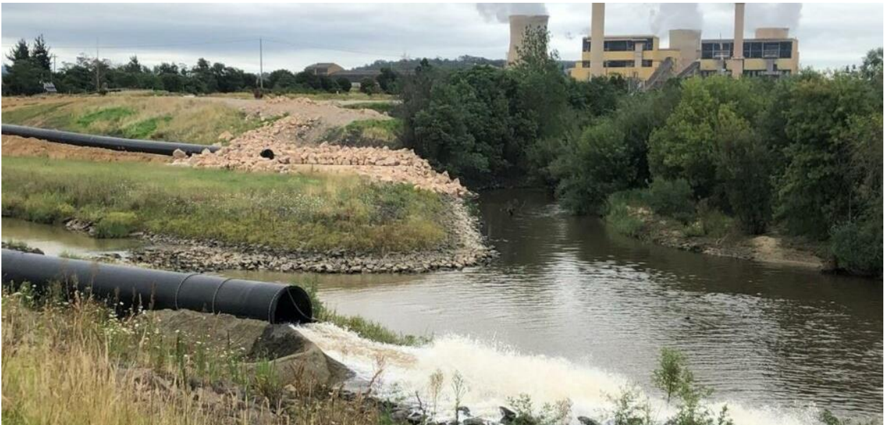
Figure 7 - 2021 A temporary river diversion (via a polyethylene pipes) was employed to support the repair of the Morwell River Diversion, picture EA website
